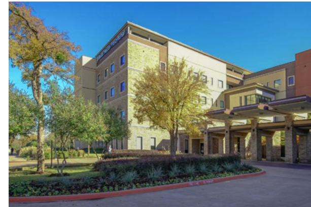
Texas Health Presbyterian Hospital
